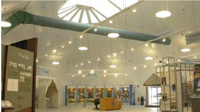
Interior of tension membrane structure
