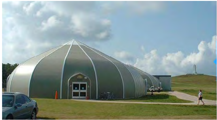
Tension membrane structure
